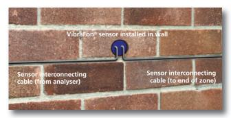
Surface mounted sensors are fixed using proprietary wall fixings and remain visible after installation. Similarly, the interconnecting cable between individual sensors in an array may be clipped directly to the face of the wall, or installed within a groove cut into the wall for this purpose.
